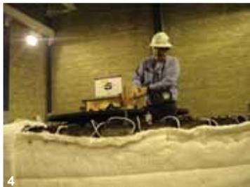
(1) Heaters applied to outer diameter (OD) of rotor rim. (2) Rim wrapped with blanket insulation. (3) Heating is carefully monitored and controlled. (4) Installing new keys in place. (At top right) Cross section of rotor shaft, hub, spider arm, rim and pole area, shown at running speed.
