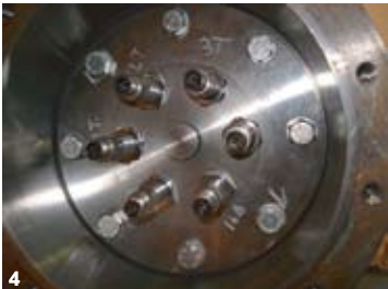
(1a) Lengthwise cross-section of hydrogen-cooled bar showing strand breakage in the interior strands. (1b) Another example of strand breakage. (2) Blocking at series connections. (3) Installation of large support rings reduces vibration. (4) Installing on-line vibration monitoring system to confirm the success of new bracing design. Graph at right shows less than 2 mils vibration, confirming the success of the retrofit.
