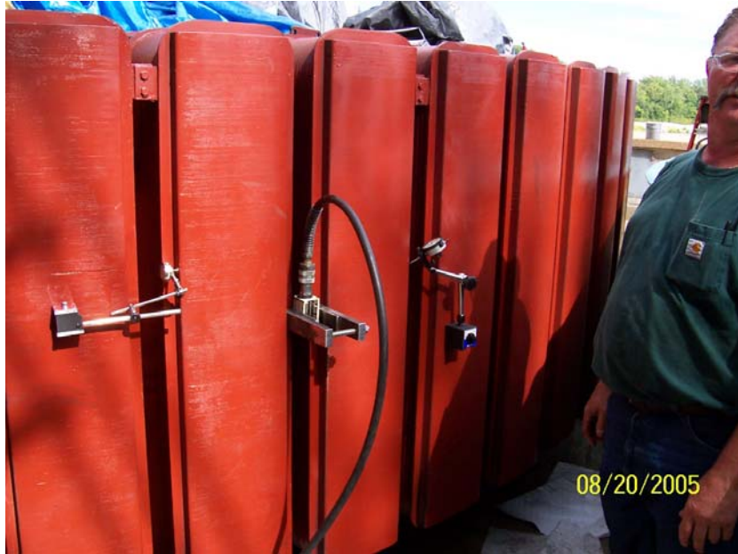
Fig. 5. Pole jacking assembly with dial indicators used to measure pole movement.
